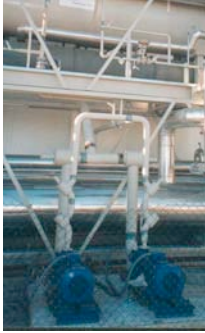
Figure 4 - Redundancy of pump and control valve
